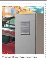
The air flow direction can easily be changed by turning the fan motor.
